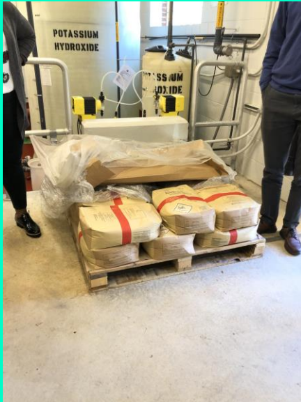
Holden Water Treatment Plant
